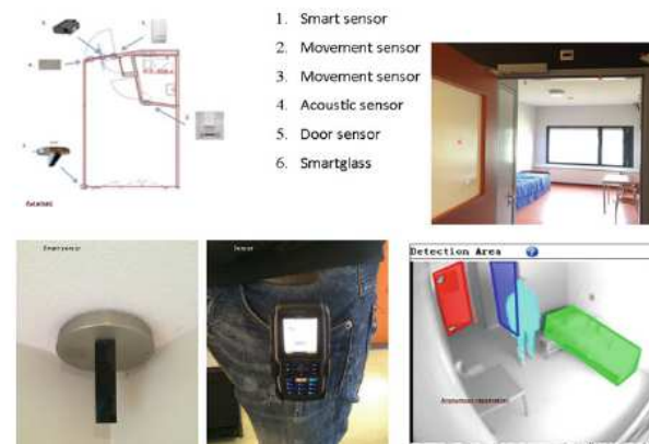
Picture 1 Technical details for the automation room
